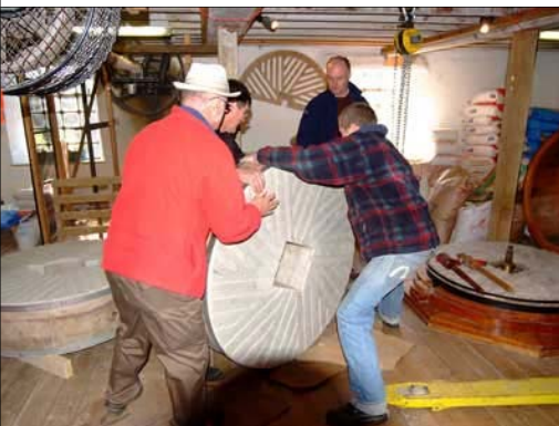
Man-handling the new millstone carefully into position and gently lower it to the floor
