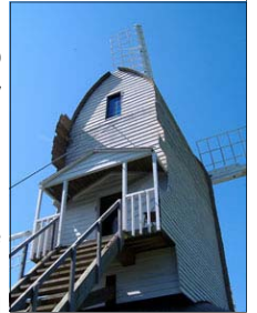
Thrigby—the wooden buck or mill body
