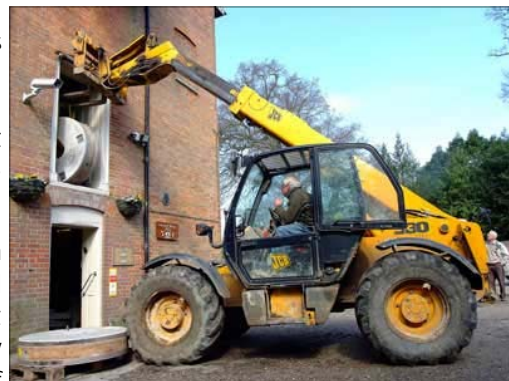
The first new millstone, the runner stone, raised to the opening of the locam and still attached to the teleporter
